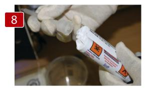
Now attach the static mixer to the cartridge. Aligning the tubes on the cartridge, gently push them together.
