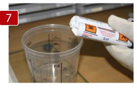
Squeeze the dispenser until both cylinders are ejecting resin. Make sure the cartridge is inclined as show in the image. (Back lower than dispensing tubes).
